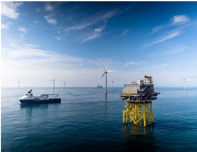
Dudgeon Offshore Wind Farm
