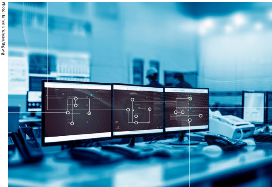
Prototype of AlarmTracker, a development project by Eldor Technology AS. The technology will increase production by helping the operator to make the right decision under abnormal situations.
