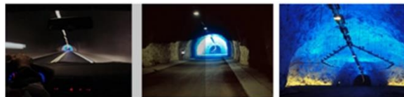
Figure 3. Rock caverns with artistic lighting effects increased safety security and reduction of monotony in the Laerdal tunnel (pictures: Dagfinn Moe, SINTEF)
